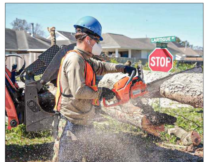
Louisiana National Guardsmen of the 159th Fighter Wing help clear roads of debris in Belle Chasse, following Hurricane Zeta, Oct. 31.
