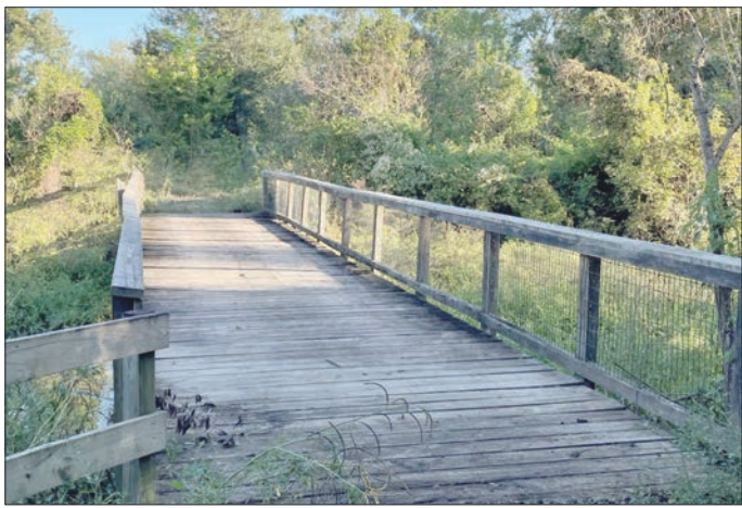
Before the bridge re-decking.
